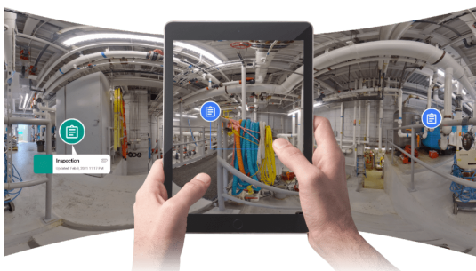
Figure 1. MEP room with annotated physical assets
